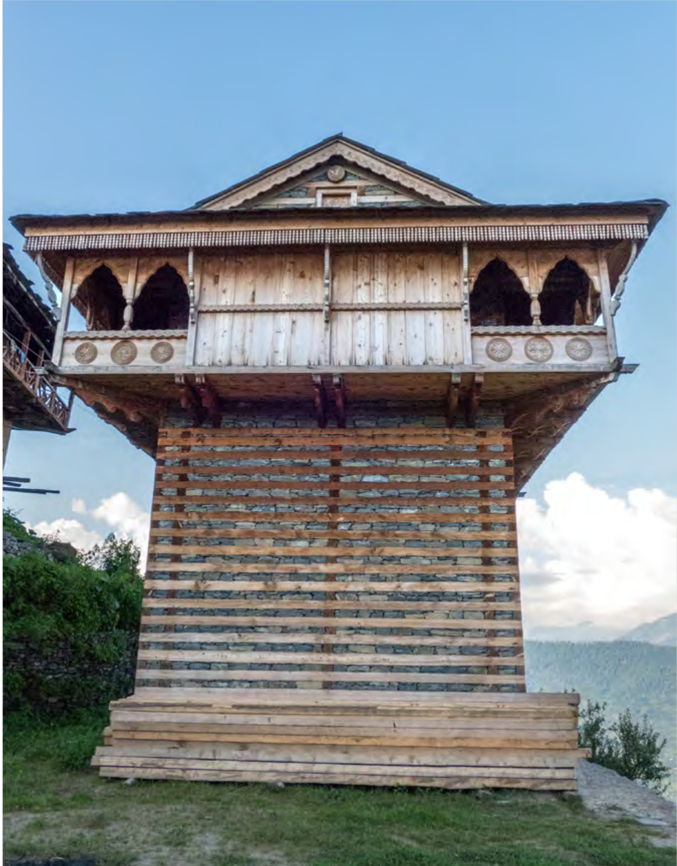
A newly constructed temple in the village of Lot dedicated to their devta, Narayan. Timber bonded structures have alternating courses of dry stone and deodar wooden beams
