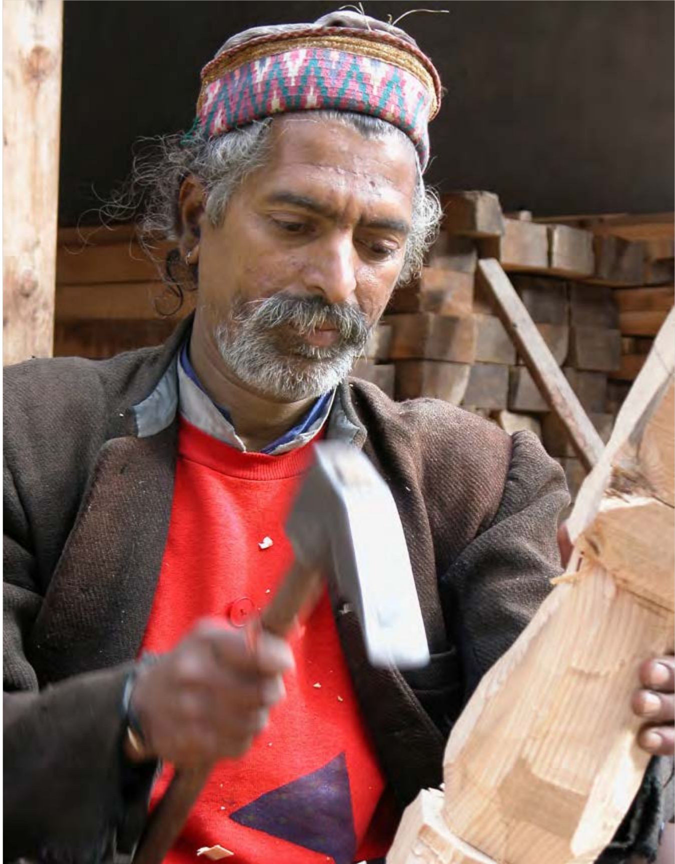
Carpenter using an adze to coarsely cut the basic form of a pillar
